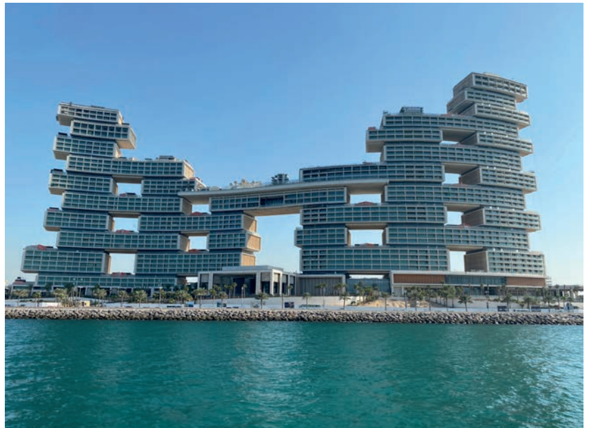
Atlantis The Royal, Dubai, United Arab Emirates Interpon D2525
